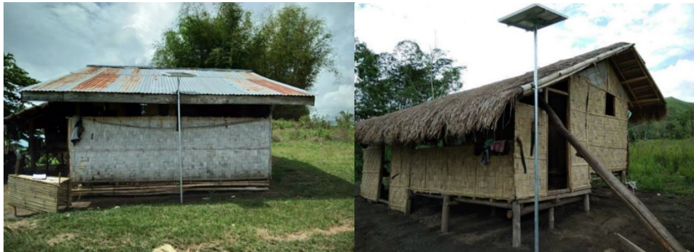
Sample Roof-side Pole mounted installation
