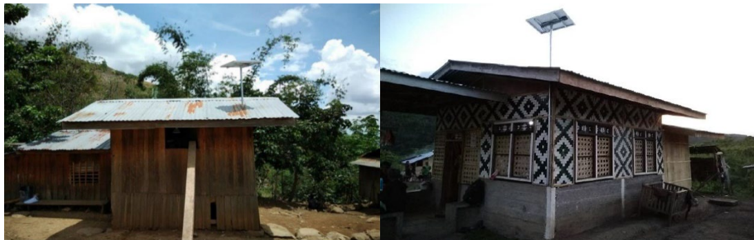
Diagram 7: Roof-through Pole mounted installations on GI roofs
