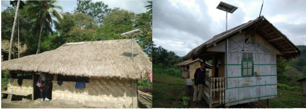
Diagram 8: Roof-through Pole mounted installations on thatched roof
